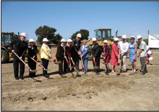
City Officials, including Mayor Bob Foster and Councilmember Tonia Reyes Uranga, homeless service agencies, and community members joined LBHDC and Century Housing for the groundbreaking of the Villages at Cabrillo's Phase III project.
